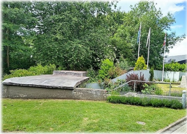
Entrance to the underground operations room
