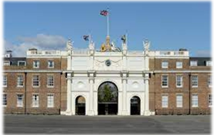
The front façade of the barracks
