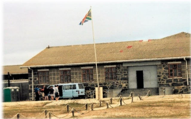
The entrance to the prison building
